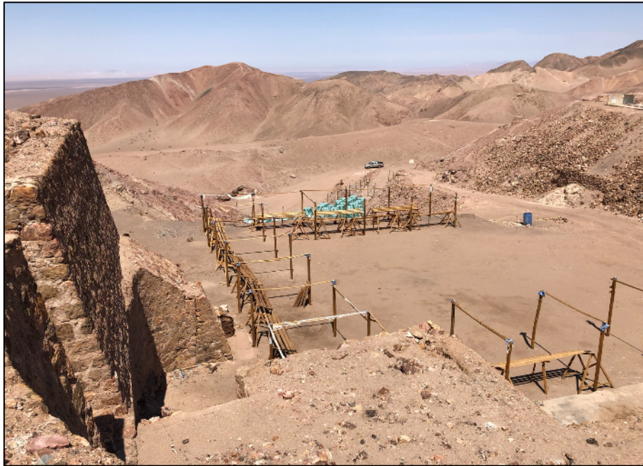
Core storage & logging facility
