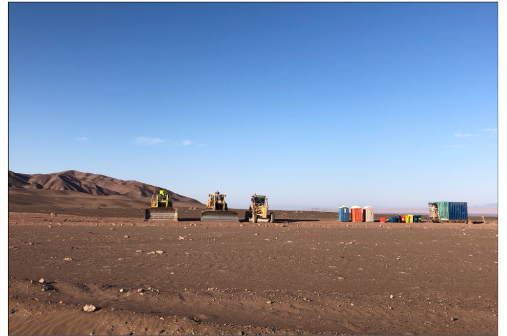
Teck water pipeline route under construction
